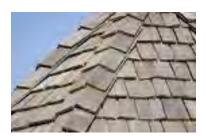
Wood shingle roofs are more easily ignitable than fire-resistant synthetic roofing materials.
